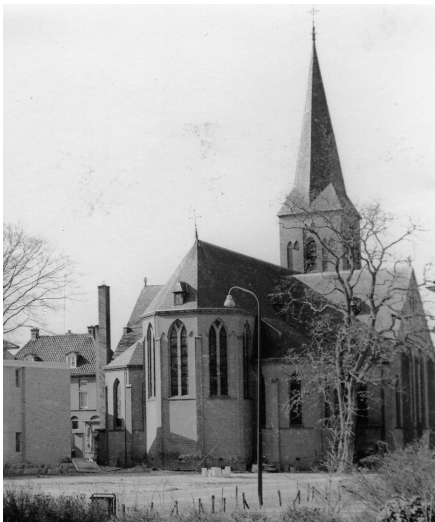
Fig. 4. The old church before demolition
