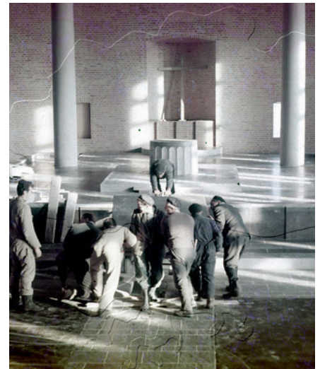
Fig. 6. Construction of the new church
